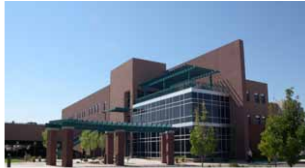
Building Oriented to Public Street
